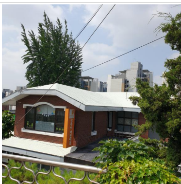
박공지붕위 COOL ROOF
